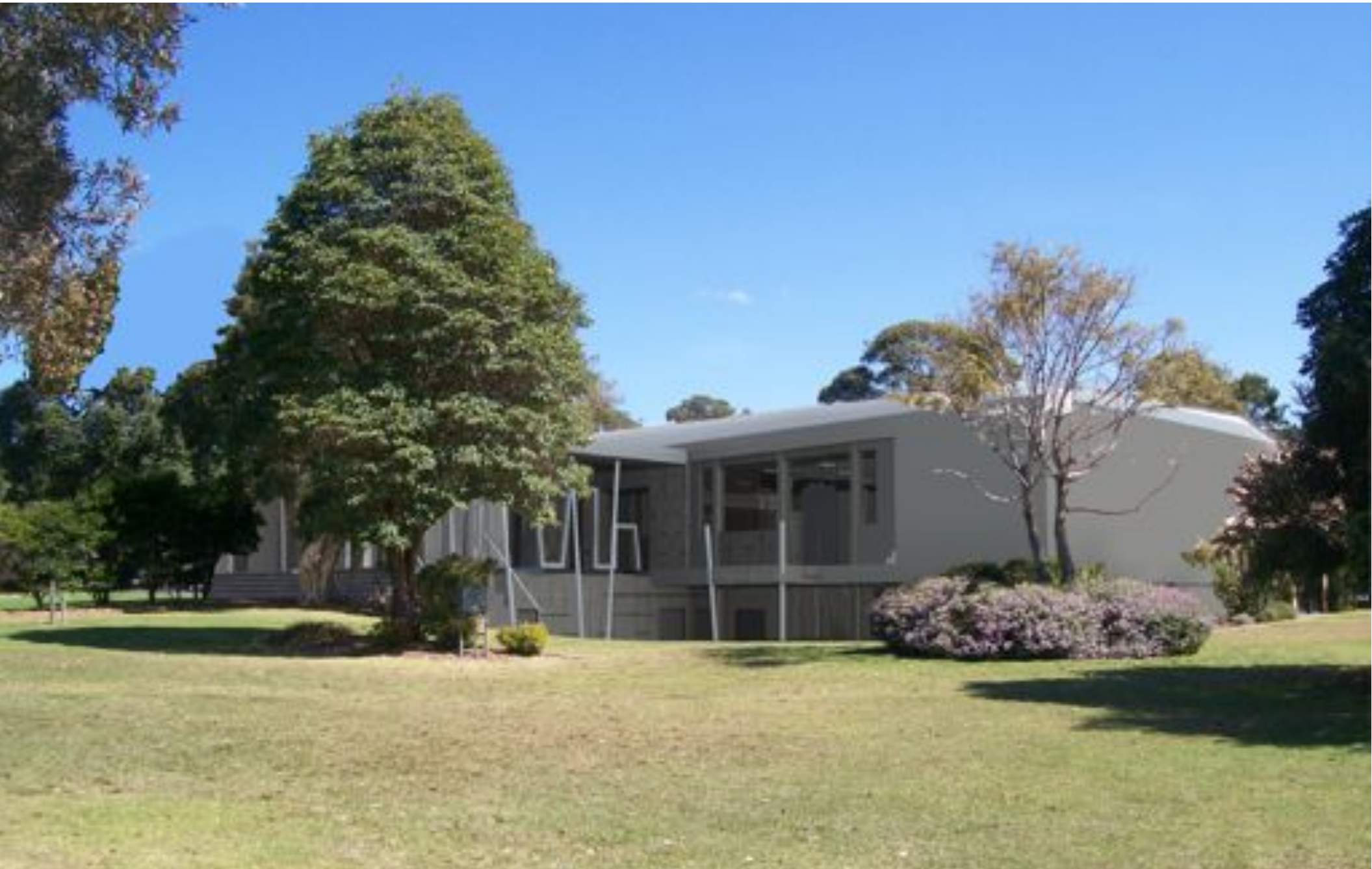
view towards north east corner PHOTO MONTAGES
